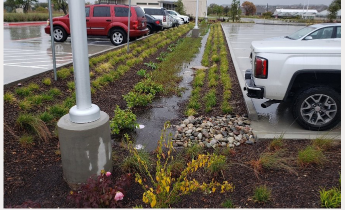
Raingarden – A shallow depression in the land constructed with stones and native plants to create ephemeral puddles to collect storm runoff.
