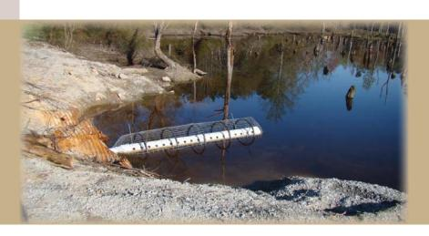
beaver build small dams across culverts, they convert the highway's foundation into a dam. These dams save the beaver significant time and effort; however, most highways are not designed to withstand the water's force, so such conditions can lead to the road's total collapse.
