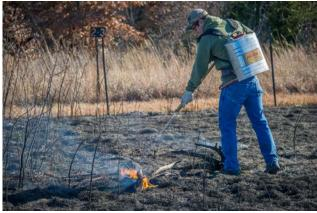
Backpack pumps can be used to lay down a wet line in areas a pumper unit may not be able to reach and to follow-up when burning from a mowed line/wet line. Backpack pumps are also very effective for suppression of small spot fires. They should be placed along the fire line where they may be needed to suppress any creeping or spot fires. (Top photo courtesy S. Coffey, bottom photo courtesy J. Weir)
