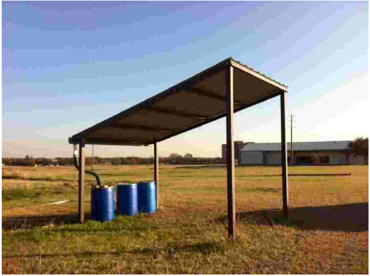
Figure 10. Rainwater harvesting and collection system
