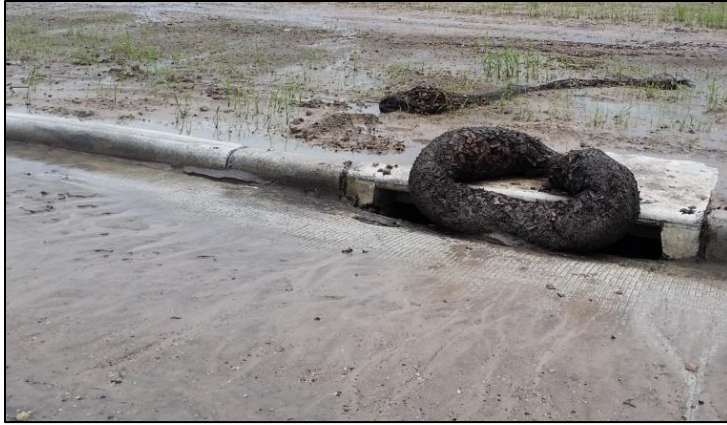
Figure 54. Example of a failing stormwater BMP; Photo taken just north of the Highland Bayou watershed
