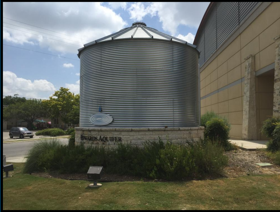
Rainwater harvesting that uses rainwater to flush indoor toilets
