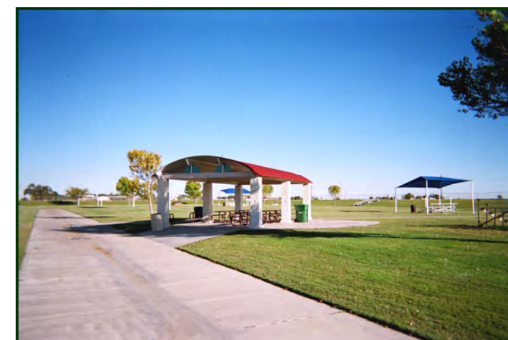
Hobbs, New Mexico – Soccer Complex built into a regional detention pond. Note pilot channels for periodic flow (also used as sidewalks), raised structures, and flood outflow structure. The entire area is contained by a fence for closure during flood events. Restrooms and concession facilities are located along the top of the adjacent levee. Stairs and ramps provide access from parking and surrounding neighborhoods.
