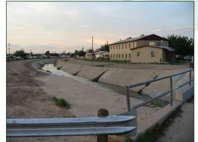
Concrete channel in the Mission Valley area.
