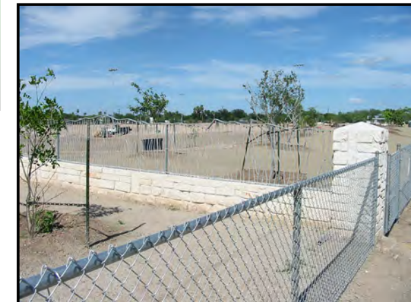
McAllen, Texas – Regional detention structure and park. During flood events, the park is enclosed by automatic gates. However, to not have such an imposing appearance, the surrounding fence is only 4' high. Ball fields will be located in the bottom of the detention area. The facility was photographed at a 90% complete stage.
