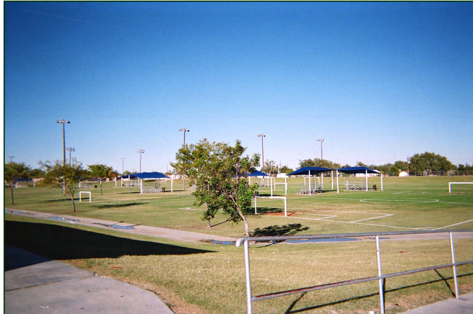
Hobbs, New Mexico – Soccer Complex built into a regional detention pond. Note pilot channels for periodic flow (also used as sidewalks), raised structures, and flood outflow structure. The entire area is contained by a fence for closure during flood events. Restrooms and concession facilities are located along the top of the adjacent levee. Stairs and ramps provide access from parking and surrounding neighborhoods.
