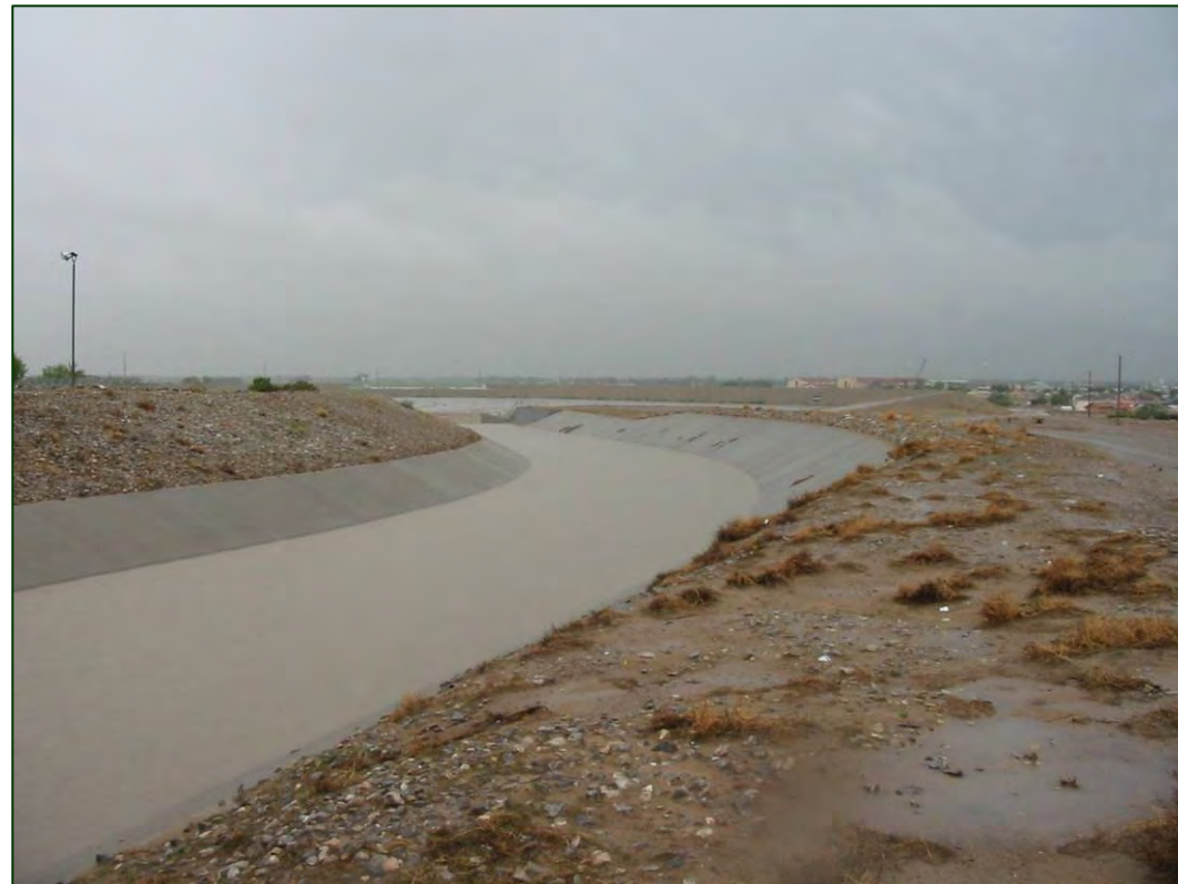
Blackie Chesser drainage channel.
