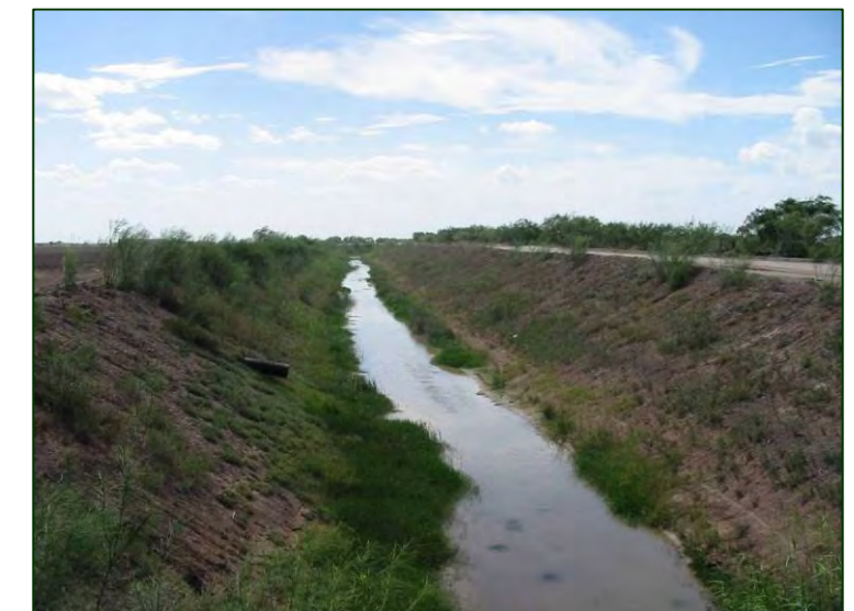
Existing earthen drainage channel in northeast El Paso.
