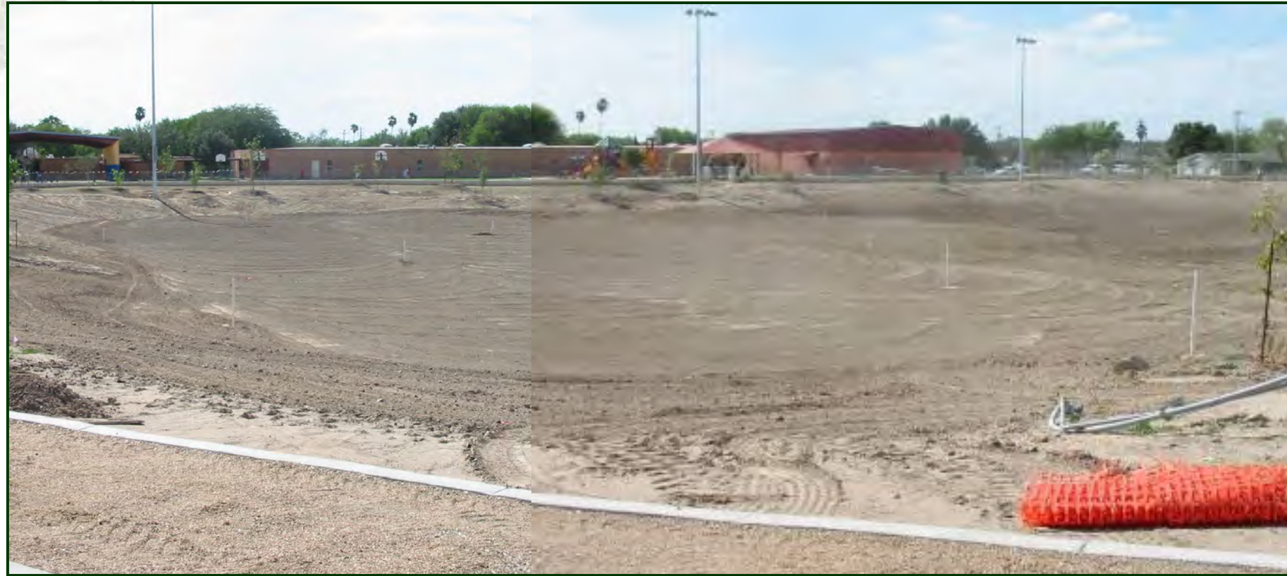
McAllen, Texas – Regional detention structure and park. During flood events, the park is enclosed by automatic gates. However, to not have such an imposing appearance, the surrounding fence is only 4' high. Ball fields will be located in the bottom of the detention area. The facility was photographed at a 90% complete stage.
