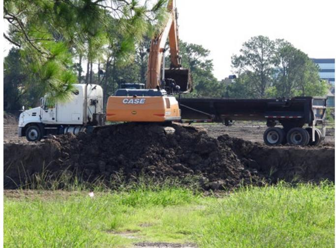
Figure 23: Hauling excess topsoil from excavation off property. Photo courtesy of Jason Miles.
