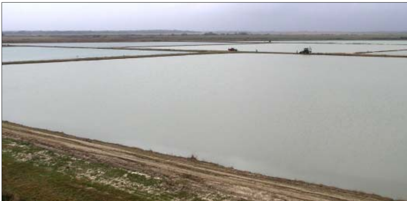
Figure 7. Completed levee ponds.
