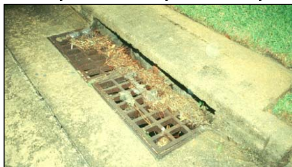
A typical storm drain with organic debris
