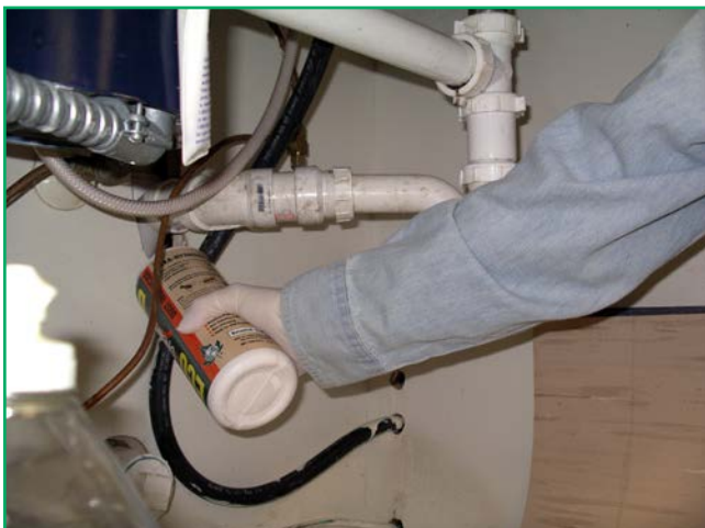
Figure 11. Applying dust to a wall void where plumbing pipes enter the wall.
