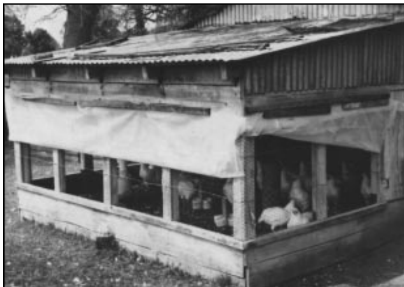
Sheds attached to existing buildings make fine facilities for growing broilers. The openings on three sides of the building provide plenty of fresh air for the birds.
