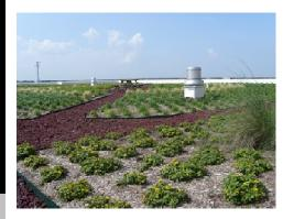
Green Roof – Roofs of buildings and other structures are impervious surfaces where water runs off. However, a roof can be designed to have a landscape on top of it. Layers of rubber membrane prevent damage to
