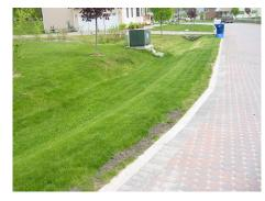
channel slows the water slightly allowing sediment to drop out. This is important because many pollutants are attached to these sediments and removing them in the swale stops them from entering our storm drain system, protecting Clear Creek and Galveston Bay.
