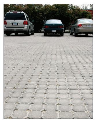
Figure 38. A porous pavement system in a shopping mall parking lot. (Photo courtesy of USDA Natural Resources Conservation Service.)
