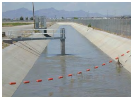
Lined American Canal Extension in El Paso
