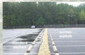
Standing Water on Standard Asphalt
