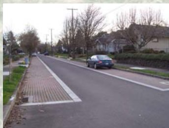
Parking Pavers Installed with Gaps
