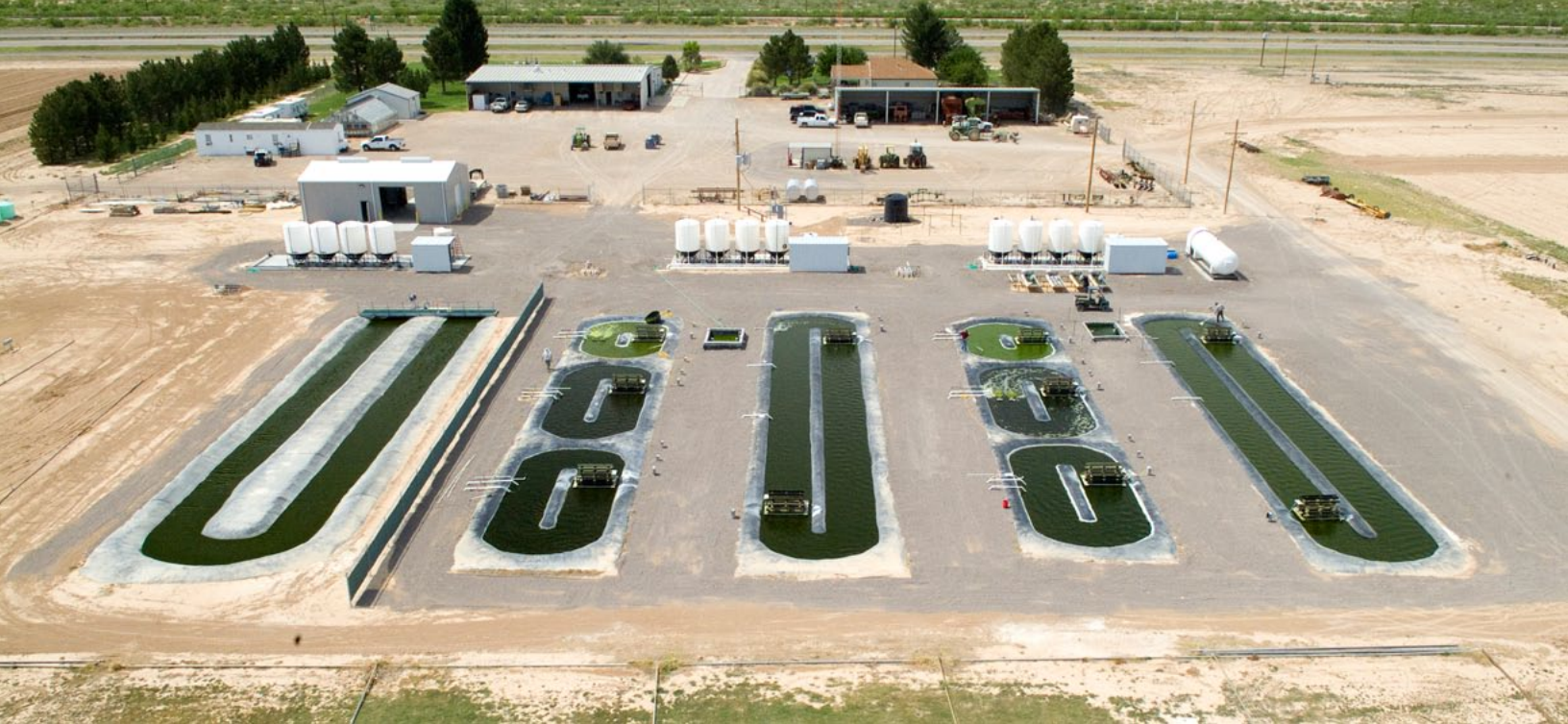
The Texas A&M Agrilife Research and Extension Center in Pecos, Texas, houses an algae demonstration facility with two sets of four ponds each, one large pond feeding into or from three smaller ponds. This facility produced a portion of the post-extraction algae residue used in the research conducted to determine the value in feeding the co-product to cattle.
