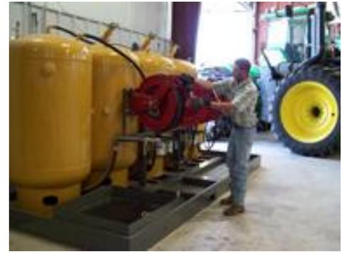
Figure 2: Portable tanks, nurse tanks, or skids (such as those provided by Sage Oil Vac, Inc. in Amarillo) are exempt from SPCC Regulations and are not counted in the total on-site fuel and oil volume. Although secondary containment is not specifically required for this class of containers, care should be taken to minimize the potential to drain fuel, oil, or waste oil into water sources. Any such discharge event is in violation of state and federal environmental laws.
