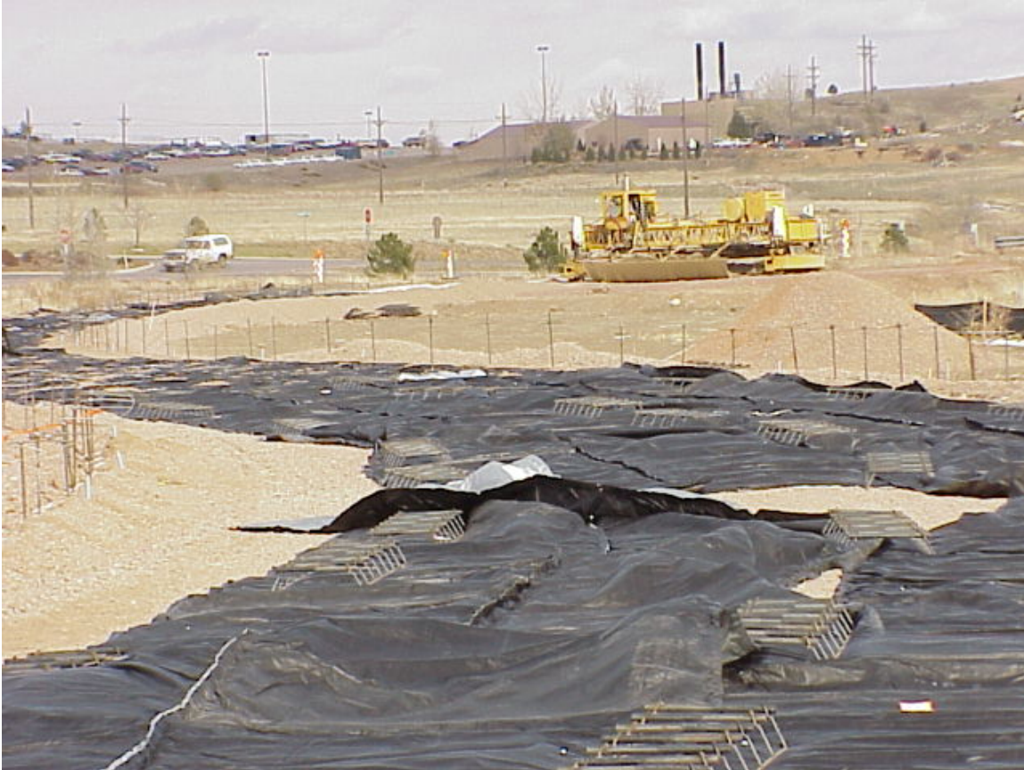
Fig. 18. Construction of a tank trail in 2000 at Cantonment II site.
